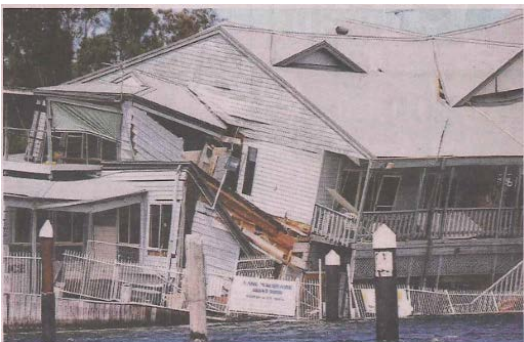
Restaurant Milano in Lake Macquarie collapsed due to soil erosion problems.
